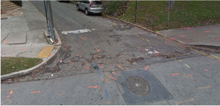
Piedmont Avenue between 10th Street & 11th Street (Ramp not flush with street and cracks in crosswalk)
