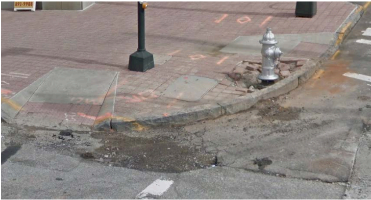
12th Street NW & Spring Street (Broken ramps)
