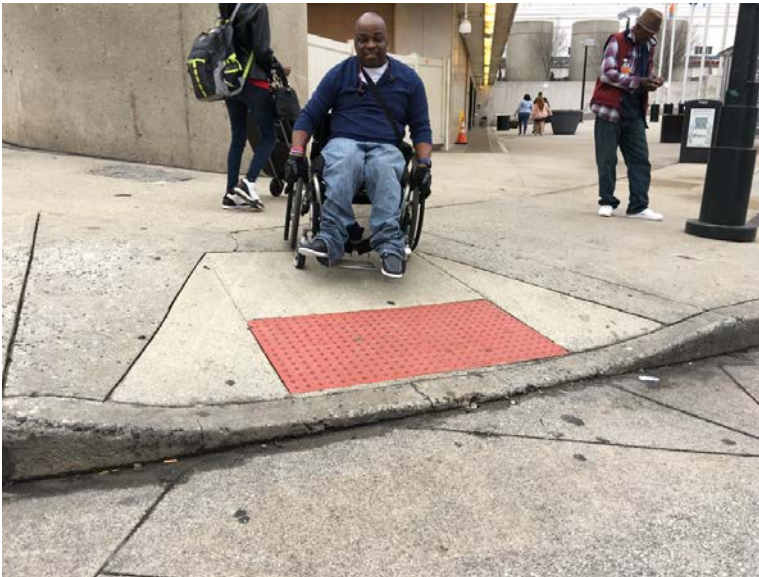
Auburn Avenue NW & Peachtree St (Ramp not flush with street & 3.6% cross slope.)
