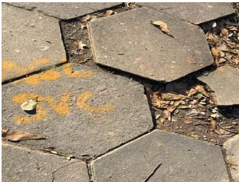
877 Edgewood Avenue (Broken, uneven Sidewalk)
