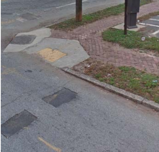
Juniper Street NE & 5th Street NE (Broken, uneven Sidewalk)
