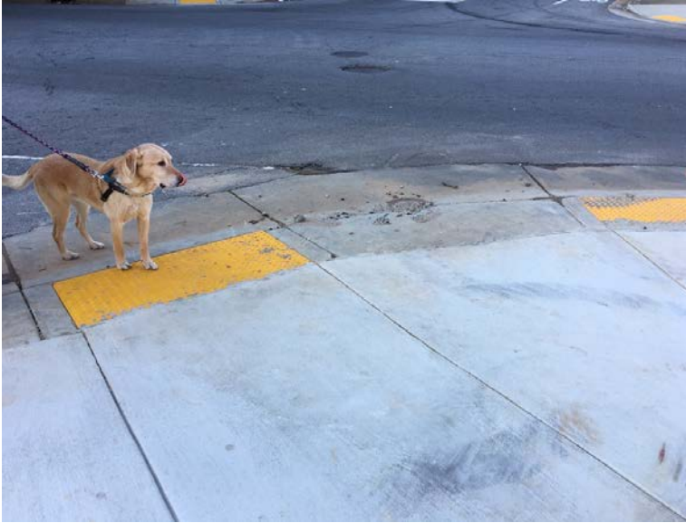
SW corner of Campbellton Rd & Lee Street (Tactile strip doesn't cover entire access from ramp)
