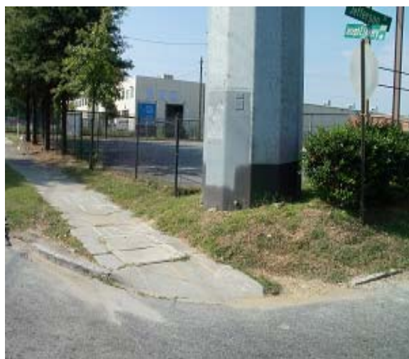
Intersection Node with Non-Compliant ADA Ramp
