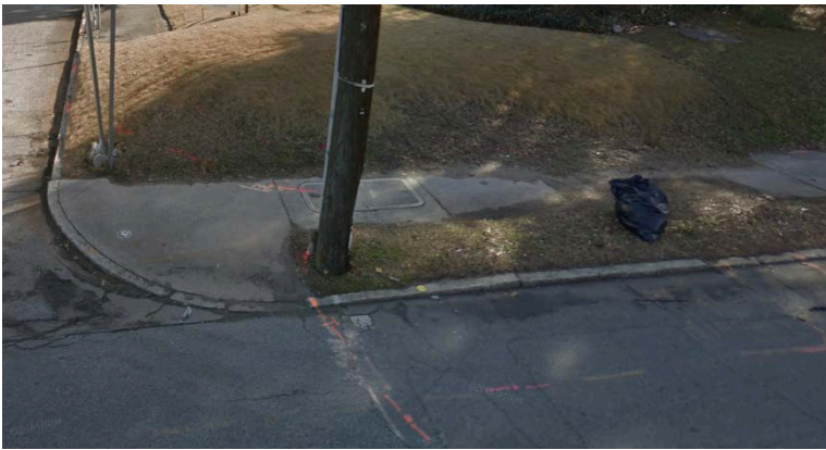
Spring Street & 19th Street NW (Broken, uneven Sidewalk)
