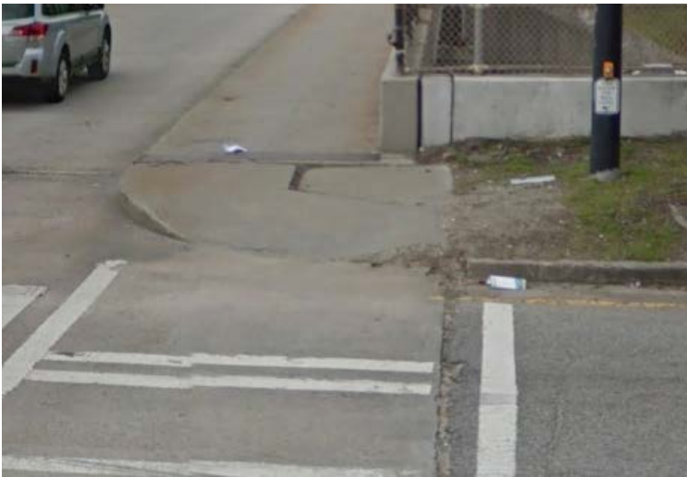
Williams Street NW (Cracks in ramp)
