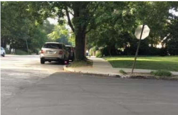
17th Street NW, east of Peachtree Street (Missing ramp)
