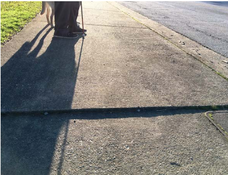
Campbellton Rd SW between Murphy Avenue and Lee St. (Broken, uneven Sidewalk)
