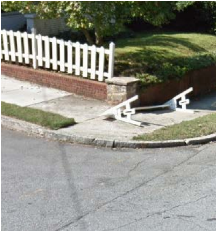
4th Street NE and Durant Place NE (Missing ramp)
