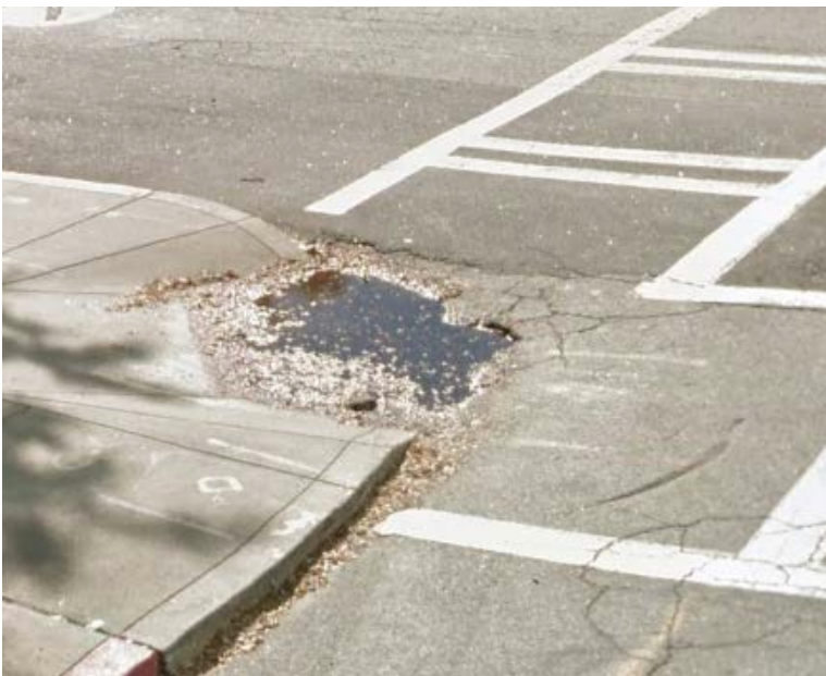
11th Street and Peachtree Walk NE (Hole at entry of ramp)
