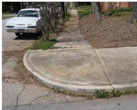
Intersection Node with Missing ADA Ramp
