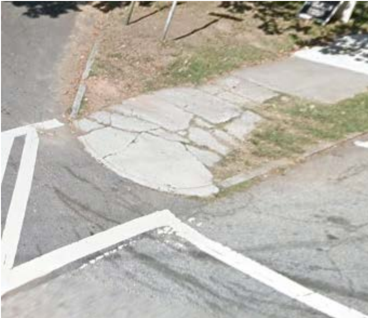
North Highland Avenue NE and Copenhill Avenue NE (Broken, uneven Sidewalk)
