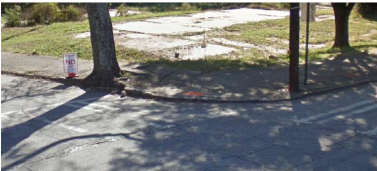
Irwin Street NE & Hilliard Street NE (Missing ramps)
