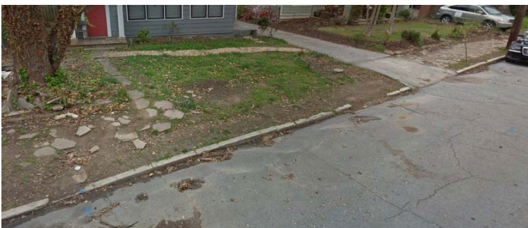
Monroe Circle NE (entire street) (Broken, missing sidewalk)
