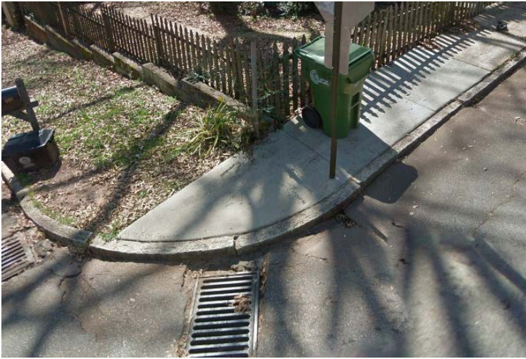
Montgomery Street & Meridian Street SE (Missing ramp)
