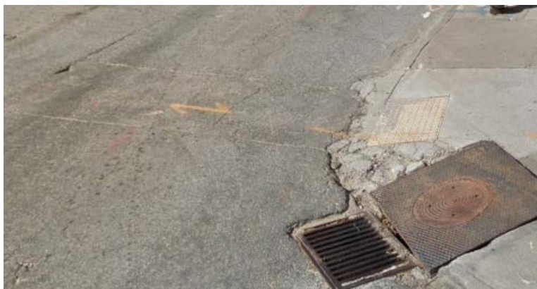
3rd Street NW (Cracks at ramp entry and no crosswalk)
