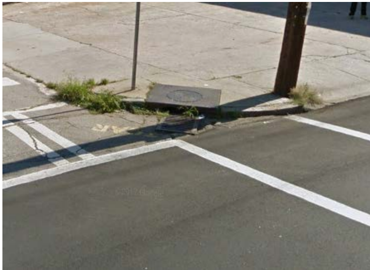
Edgewood Avenue at William H Borders Sr Drive (Missing ramps)
