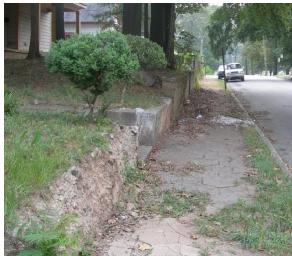
Deteriorated & Non-ADA Compliant Sidewalk
