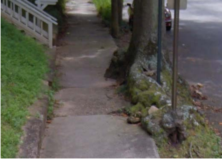
Atlantic Drive NW & 11th Street (Broken, uneven Sidewalk)
