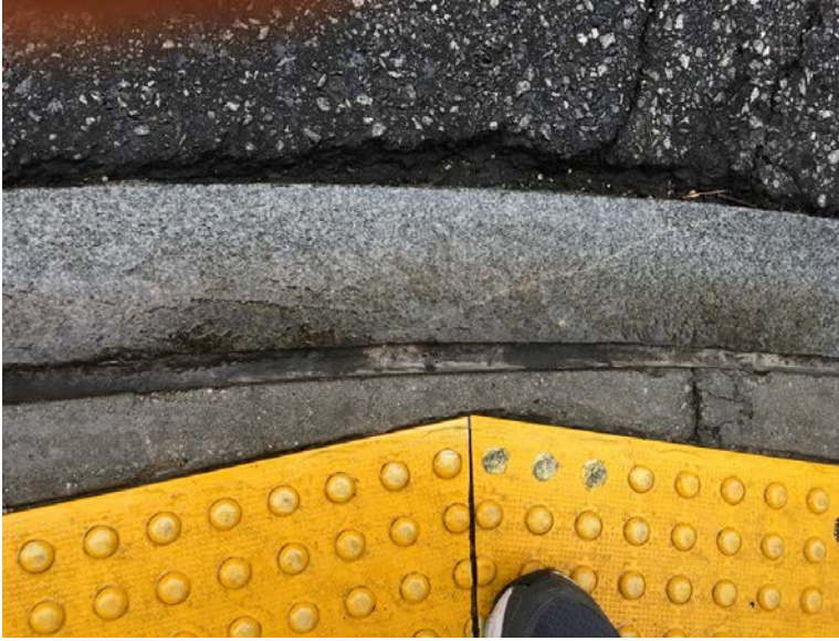
45 Marietta St, ramp at SE corner - Forsyth Intersection (Not flush with street)
