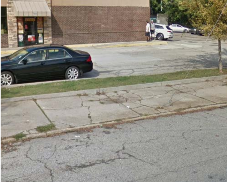
Piedmont Avenue north of Ponce de Leon Avenue NE (Broken, uneven Sidewalk)
