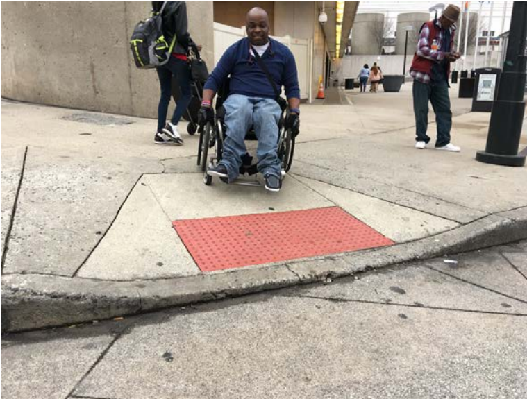
Auburn Avenue NW & Peachtree St (Ramp not flush with street & 3.6% cross slope.)
