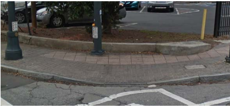
Peachtree Street NE & Ralph McGill Boulevard NE (Cracks in crosswalk, narrow passage)
