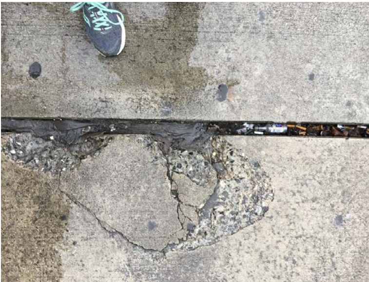
East side of Forsyth St between Marietta St and Five Points Station (Broken pavement and gap between sidewalk slabs)
