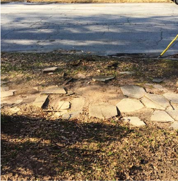
Adjacent to green space across the street from 846 Euclid (Broken, uneven Sidewalk)
