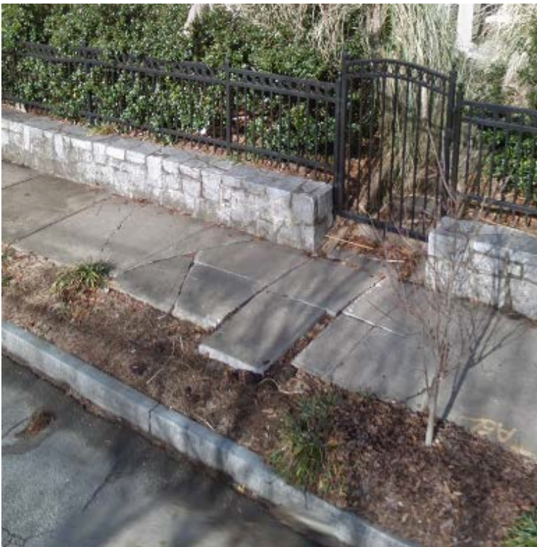
Montgomery Ferry Drive NE between Flagler Ave NE & Monroe Drive NE (Broken, uneven sidewalk)
