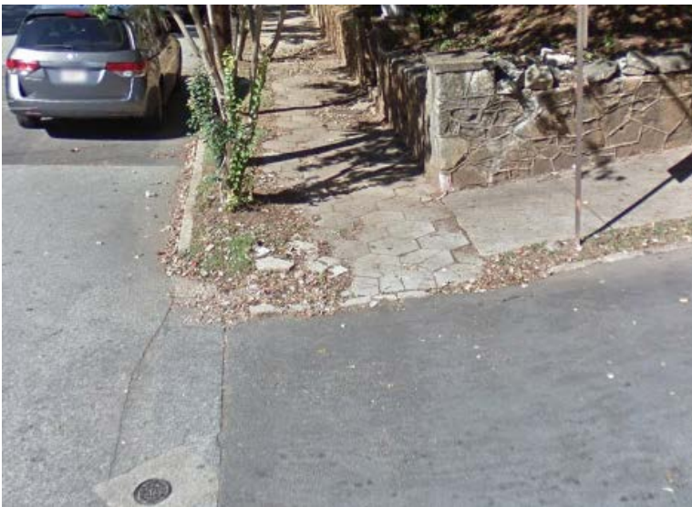
Todd Road NE & Highland View NE (Broken, uneven Sidewalk)
