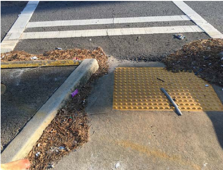
Island at NW corner of Dill Avenue & Lee St. (No flare between ramp and flat pavement)
