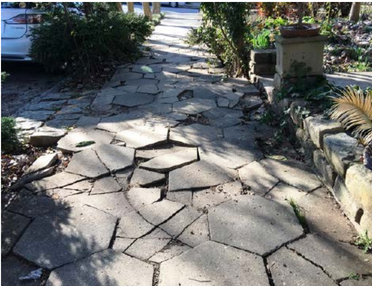
752 Dixie Avenue (Broken, uneven Sidewalk)
