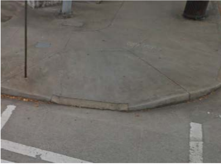
Courtland Street NE and Ralph McGill Boulevard NE (Ramp not flush)
