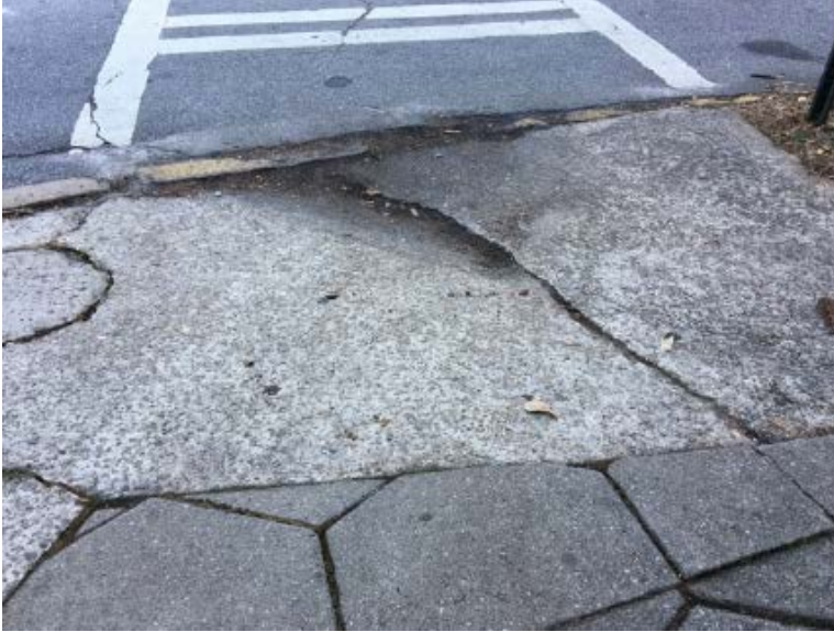
SW corner of Edgewood Avenue & Hurt Street (Cracks in ramp)
