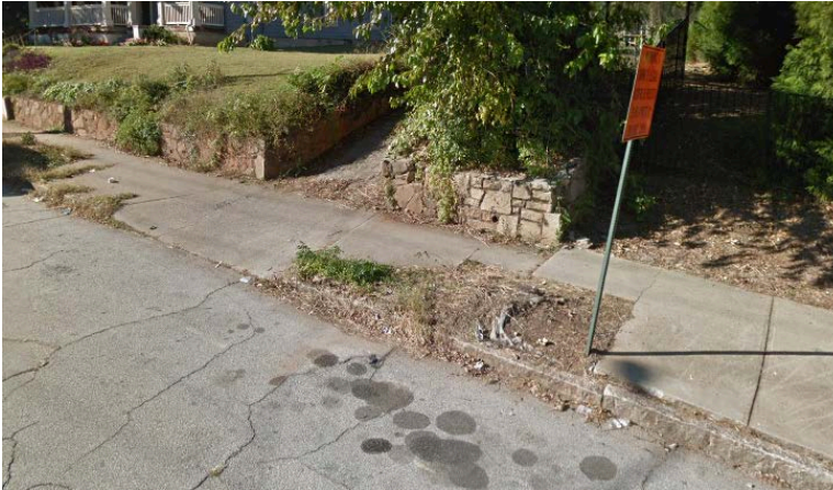
Irwin Street NE between Jackson Street NE & Hilliard Street NE (obstructed Passage and uplifted concrete slab)
