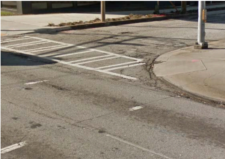
18th Street & Spring Street (Improper crosswalk markings)
