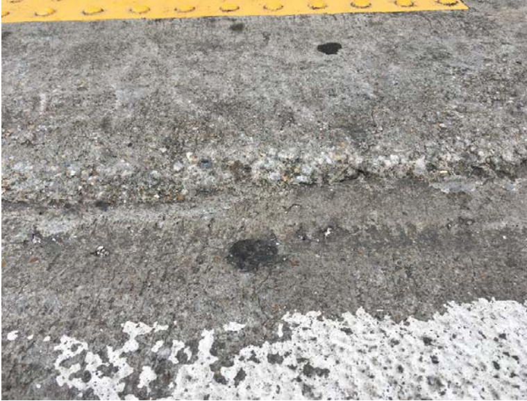
Wall St and Peachtree ST, SW corner (Ramp not flush with street)
