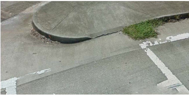
Courtland Street NE and Ralph McGill Boulevard NE (Ramp not flush with crosswalk)
