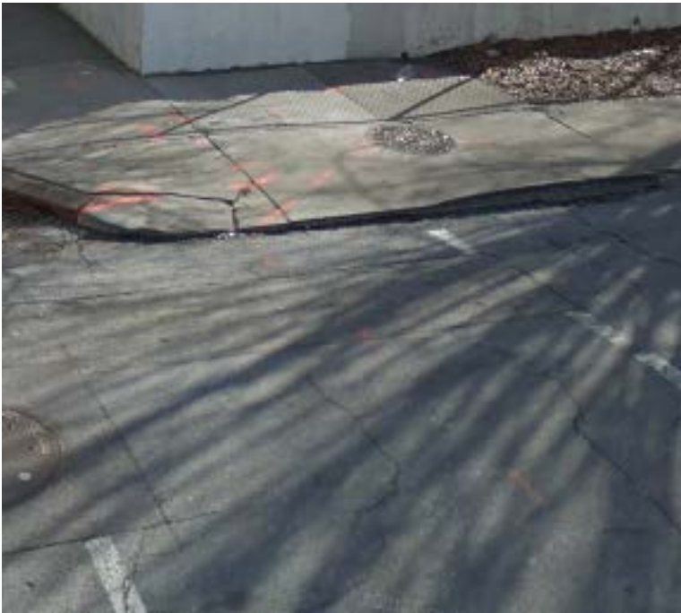
3rd and Spring Street NW (Missing ramp)
