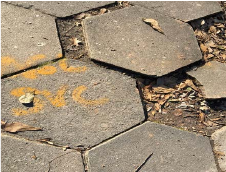
877 Edgewood Avenue (Broken, uneven Sidewalk)
