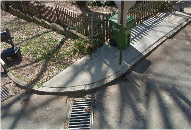
Montgomery Street & Meridian Street SE (Missing ramp)
