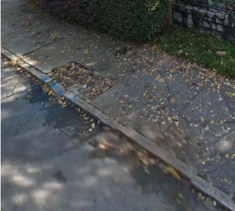
Piedmont Avenue & 4th Street NE (Broken, uneven Sidewalk)
