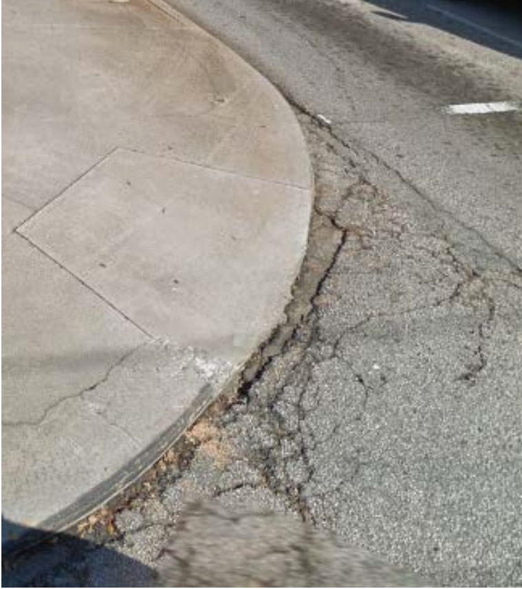
18th Street and Spring Street (Hole at ramp entry)
