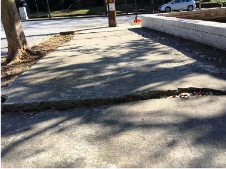
892 Edgewood Avenue (Broken, uneven Sidewalk)
