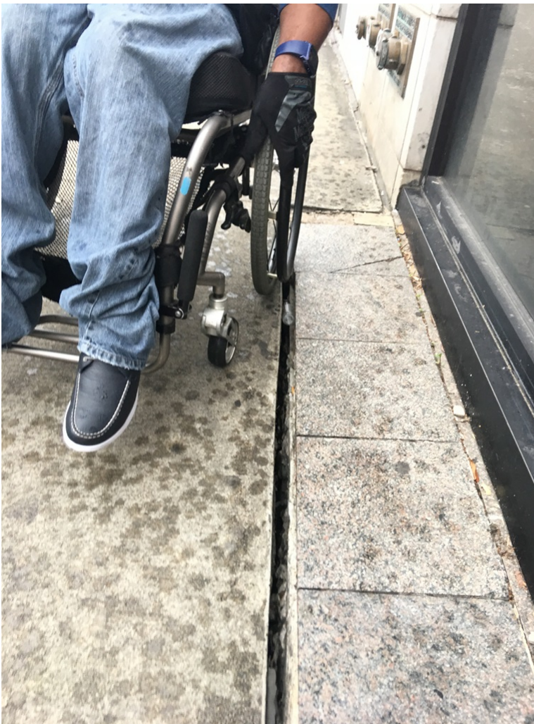
Across from 15 Peachtree St (Gap in sidewalk slab)
