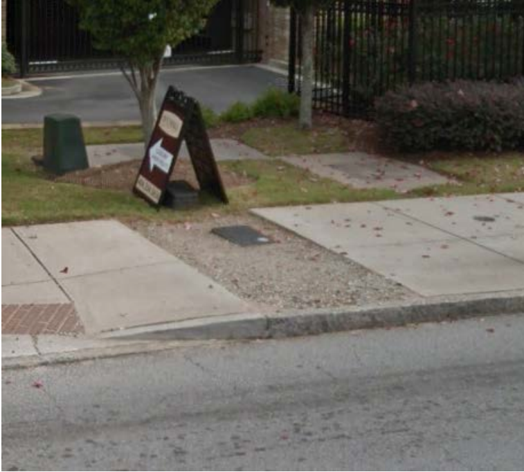
Piedmont Avenue between Ponce de Leon Avenue NE & North Avenue (Missing sidewalk panel)
