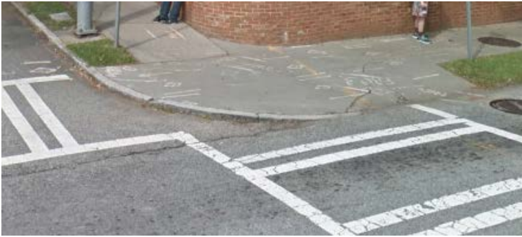
Atlantic Drive NW & 10th St NW (Missing ramp)
