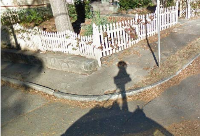
4th Street NE and Durant Place NE (Missing ramp)
