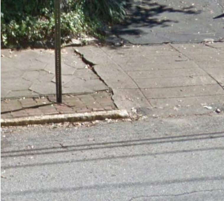
North Highland Avenue NE (Disjointed sidewalk)
