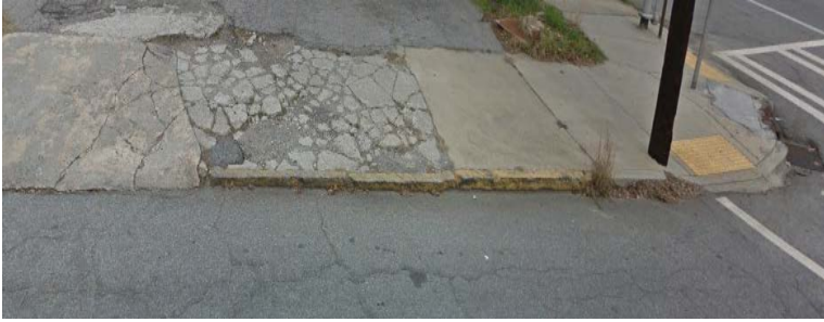
Renaissance Parkway & Courtland Street NE (Broken, uneven Sidewalk)
