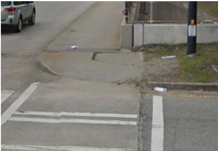
Williams Street NW (Cracks in ramp)
