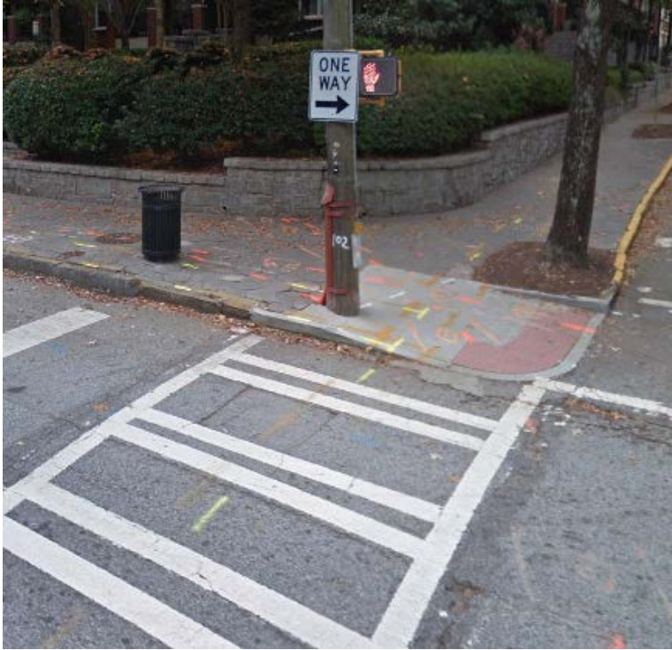
Piedmont Avenue NE & 7th Street NE (Ramp in need of repair)
