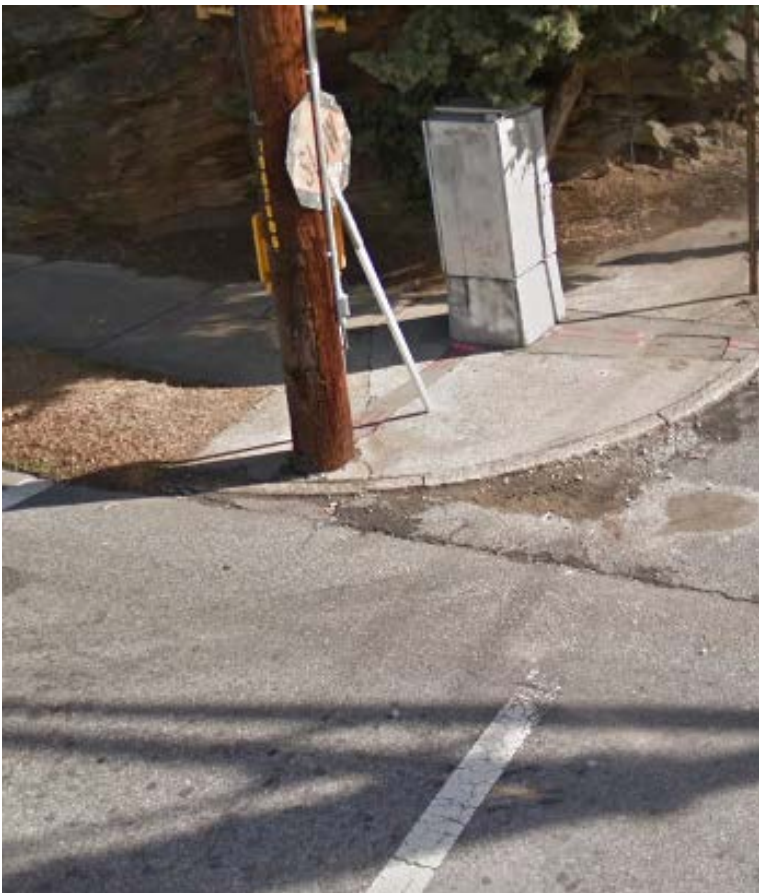
18th Street NW and Spring Street (Obstructed ramp)
