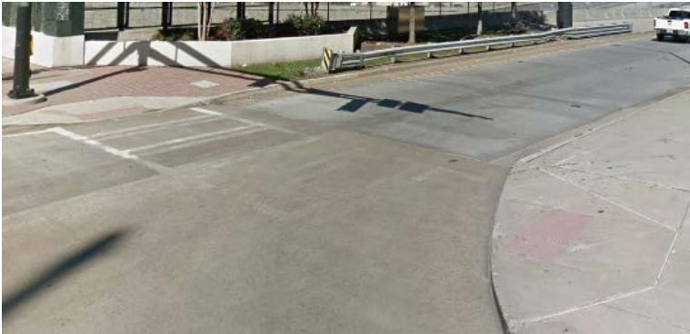
Williams Street & 14th Street NW (Improper crosswalk markings)
