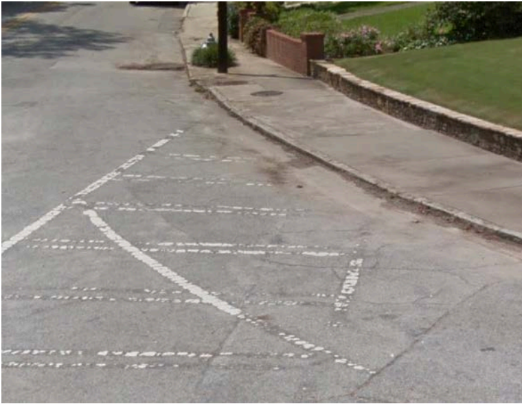
Montgomery Ferry Drive NE & Polo Drive NE (Missing Ramp)
